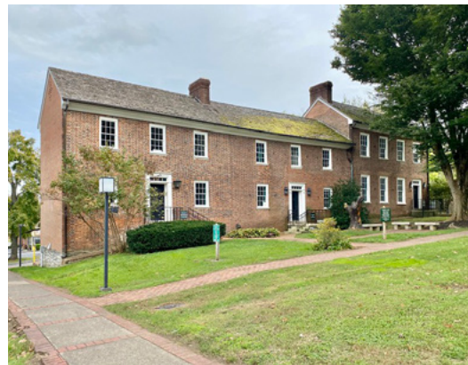
Brick Schoolhouse, c. 1820
