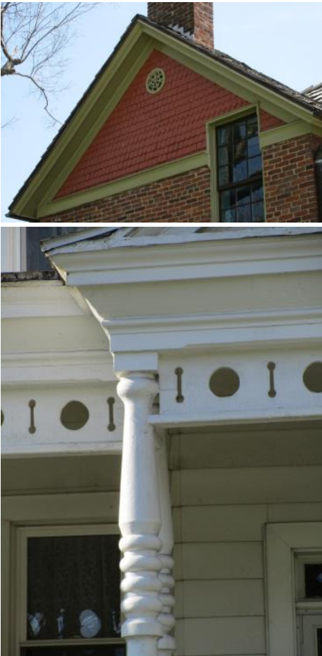
Wood is used in both simple and complex details in the historic overlay district, from decorative shingles to turned porch posts.
