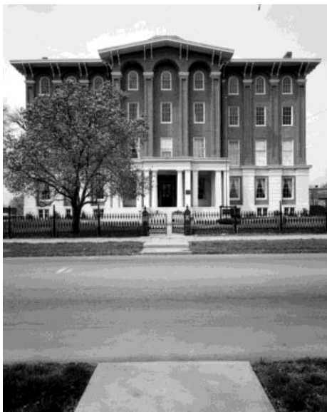
Jacobs Hall, Kentucky School for the Deaf. Historic American Building Survey, Library of Congress, Prints and Photographs Division.
