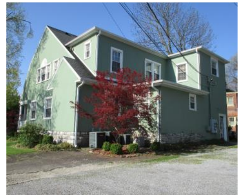
Locating modern mechanical equipment and utilities to side or rear elevations and/or screening with vegetation, as demonstrated above, is strongly encouraged.
