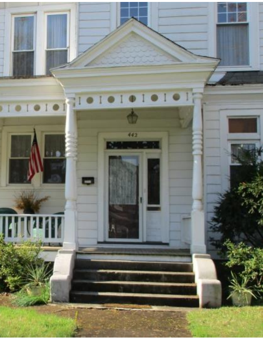
Storm doors that provide a full view of the primary door are the most appropriate design choice.
